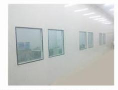
**WALL PANEL** partitions are a composite construction of two skin of PPGI or SS304 over an GI with powder coated frame work with a sealed and insulated interior. Standard panel dimensions are 1200x3000mm an overall thickness ranges of 100/80/60 mm. The self-supporting internal walls are constructed with an interior GI frame work. The Partition seams are sealed by silicone with a perfectly flush finishing. PUF insulation material is sandwiched between the two skin layers PPGI or SS304
